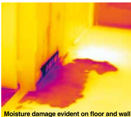
Moisture damage evident on floor and wall
